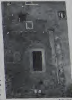
Fig. 12. SC. Quatre Corneils. Field shows the remains of arches and wall.
